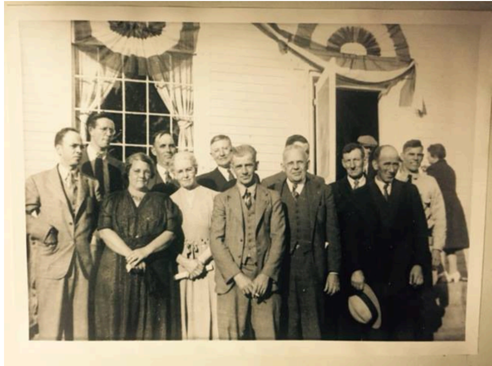
Courtesy of Vermont Electric Cooperative .
